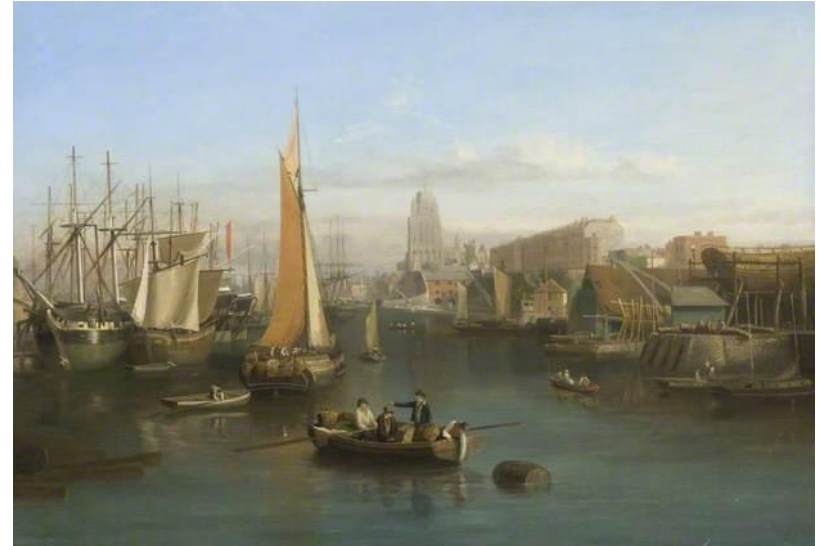
St Mary Redcliffe and Redcliffe Parade from Prince Street Bridge
